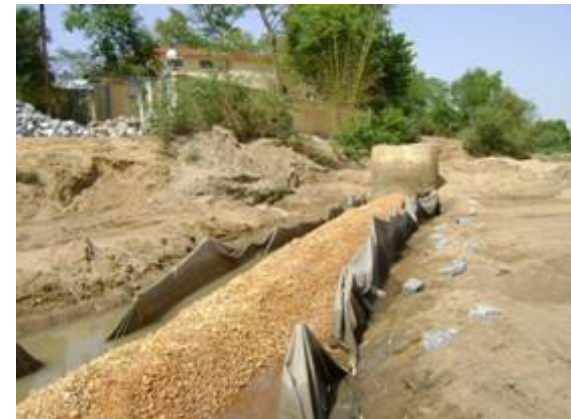
Installing geotextile wrapped around pipes
