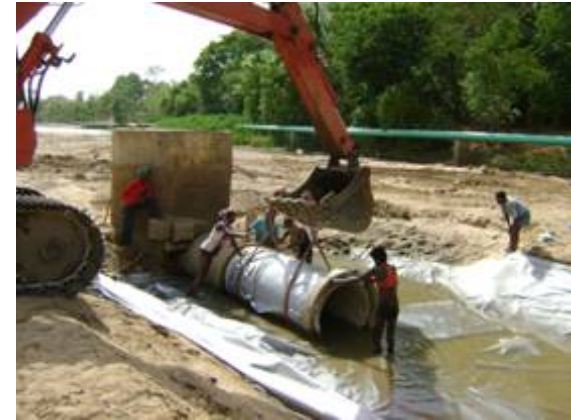
Installing geotextile wrapped around pipes
