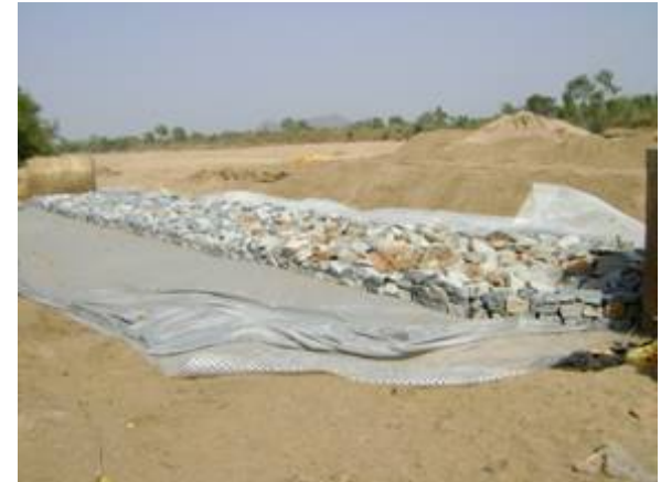
Boulders for gabion mattress
